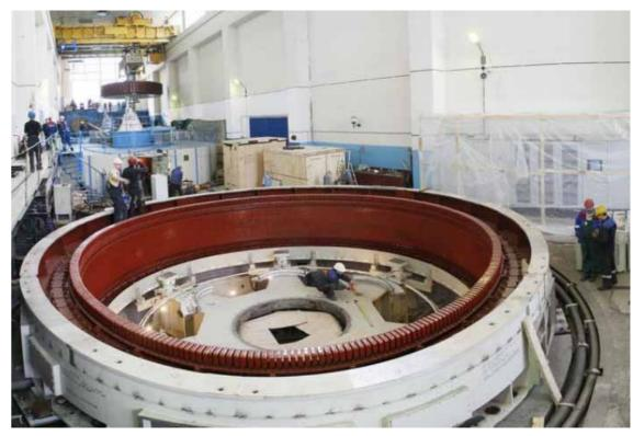
Fig. 26. Installation of a rotor of a Hydropower Unit at Lesogorskaya HPP
