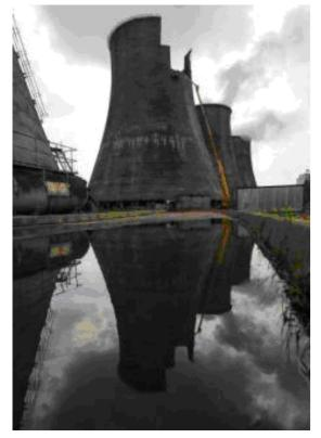
*Fig. 21. TPP-16: Disassembly of Cooling Tower No. 2*
