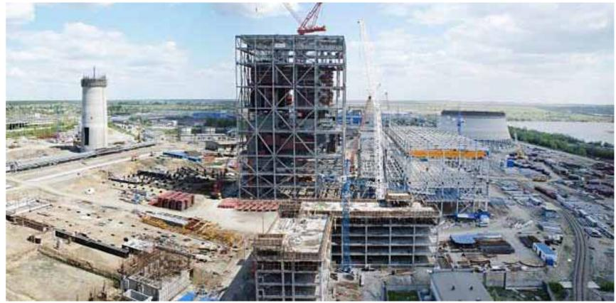
Fig. 33. Construction of a new coal dust generation unit at Troitskaya GRES
